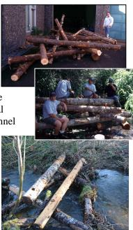
as riparian protection and silvicultural solutions begin to take hold. Unfortunately, functional LWD is difficult to procure in the quantities required, and is very expensive to transport and place due to its weight. The object of this paper is to introduce an engineered log jam structure that is easy to transport and install by citizen volunteer and conservation crews.
