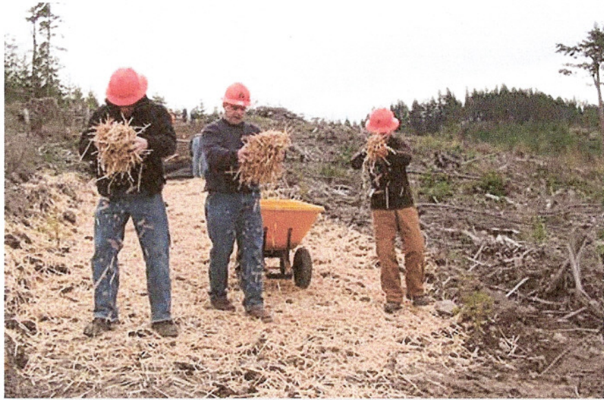
WOODSTRAW™ BEING APPLIED FOR EROSION CONTROL
