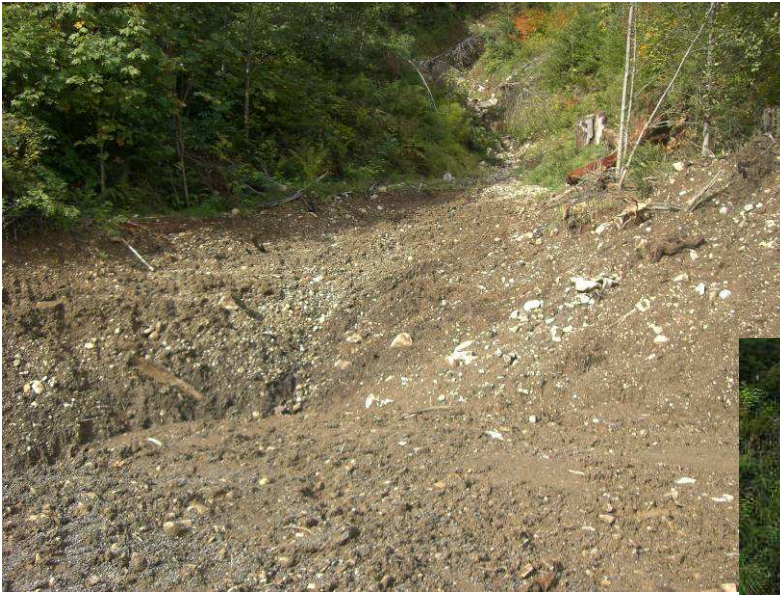
Roadside Culvert Repair
