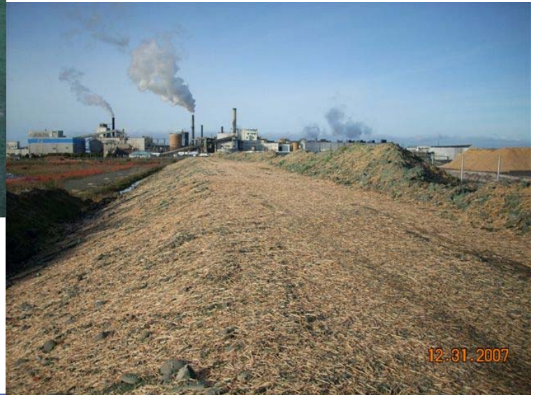
After WoodStraw™ Application Over Hydroseed 250 regular bales
