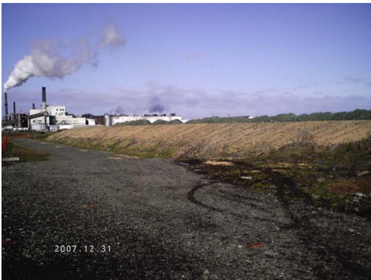
After WoodStraw™ Application Over Hydroseed 250 regular bales
