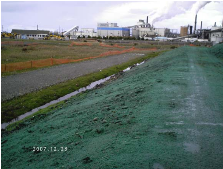
Before WoodStraw™ Application (Hydroseed)
