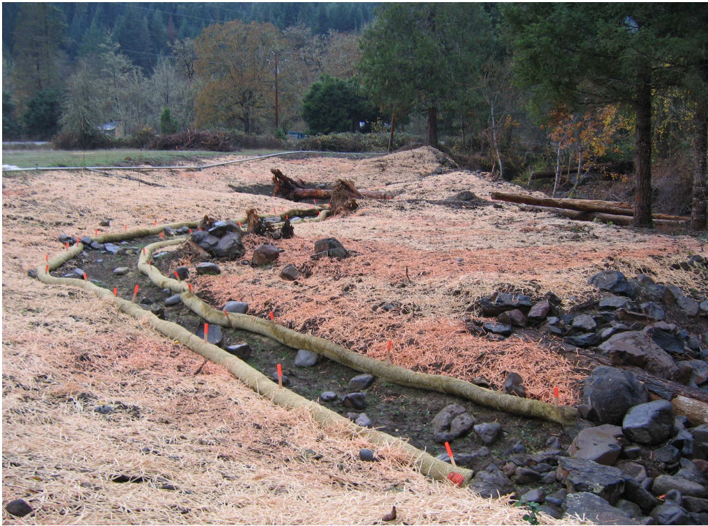
In-stream restoration project using WoodStraw™ for erosion control
