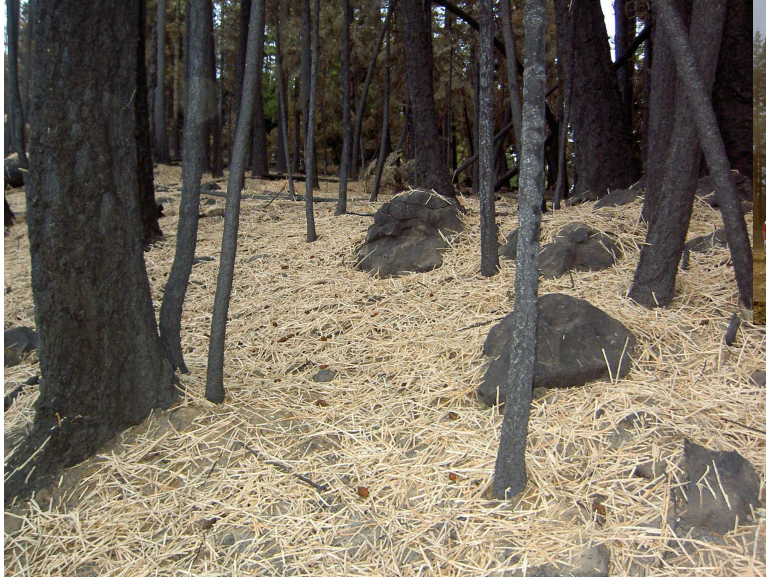
Area of helimulching with WoodStraw™ wood-strand erosion control mulch.
