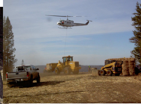
Area of helimulching with WoodStraw™ wood-strand erosion control mulch.
