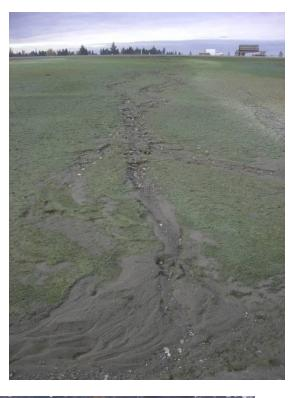
Significant erosion and sediment movement on hydroseed and blankets.
